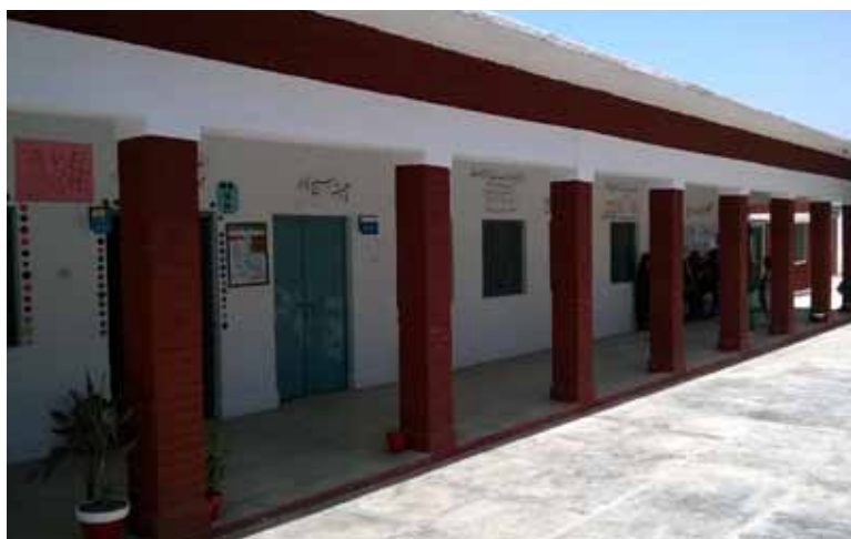
School Rehabilitated under Telenor School Rehabilitation and Improvement Project, District Nowshehra
